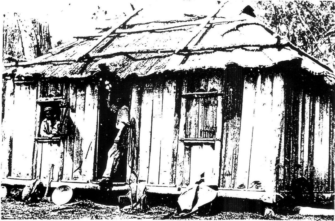
Anthony, Henry and Ned Whitten first lived in slab huts like this.
