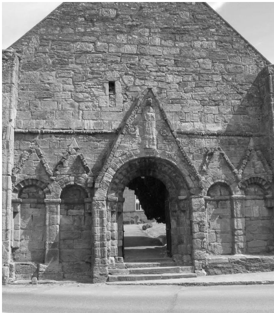
Old West Gable
